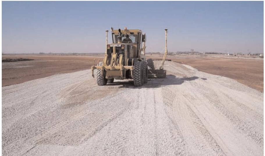
Completed sub ballast installation on Mirafi® HP570.
