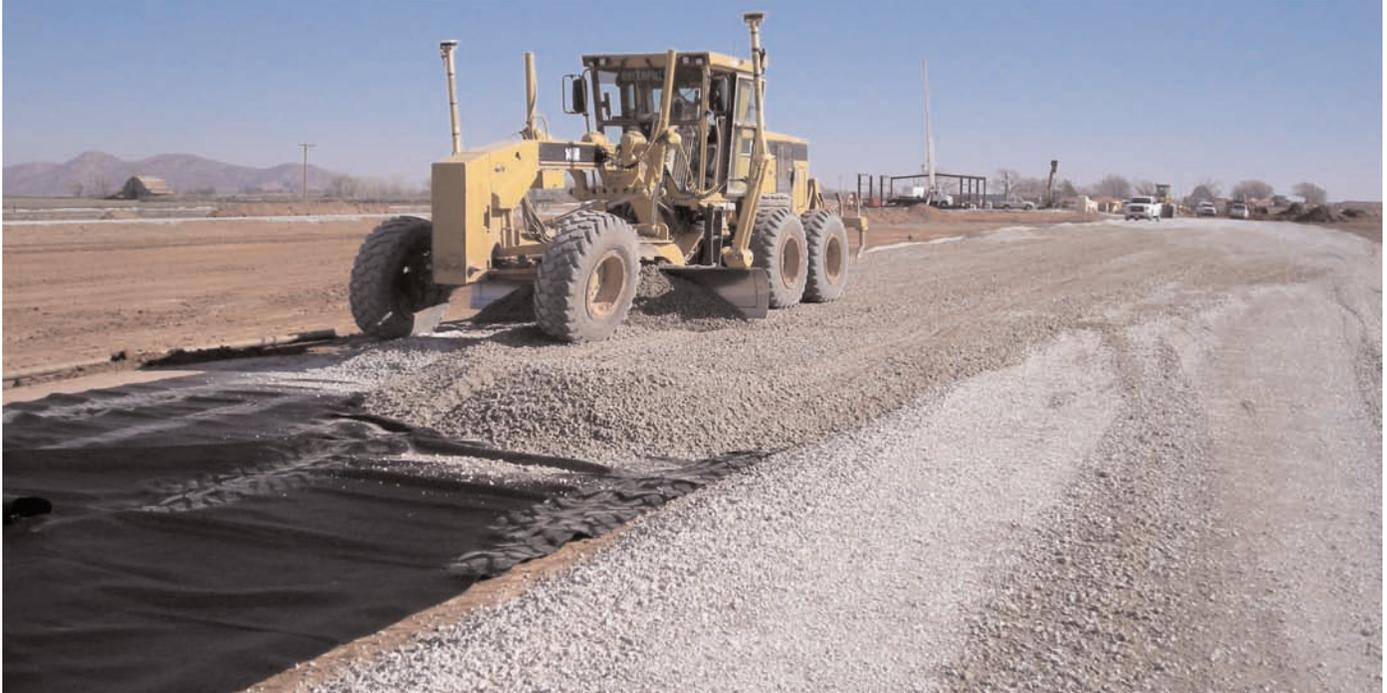
Backfilling of sub ballast on Mirafi® HP570.
