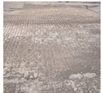
Pavement milled and prepped for leveling.
