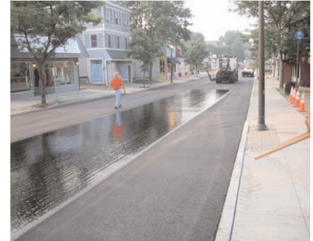
Installing in liquid asphalt ensures the mat will provide necessary moisture protection from water intrusion.
