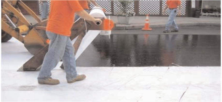
Installing in liquid asphalt ensures the mat will provide necessary moisture protection from water intrusion.
