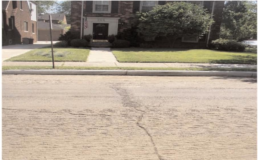
Photo taken in July 2006 as part of construction preparation of the asphalt wearing course showing fatigued pavement transverse cracking. Milled curb lanes were done to improve crown and slope corrections prior to paving.
