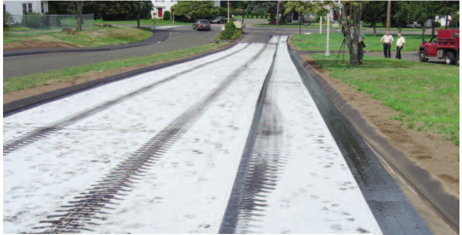
Figure 4: TruPave® installed over roadway...ready for chip seal installation.
