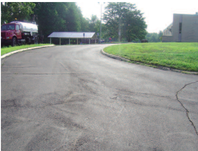
Figure 1: Typical pavement conditions prior to TruPave® with chip seal application.
