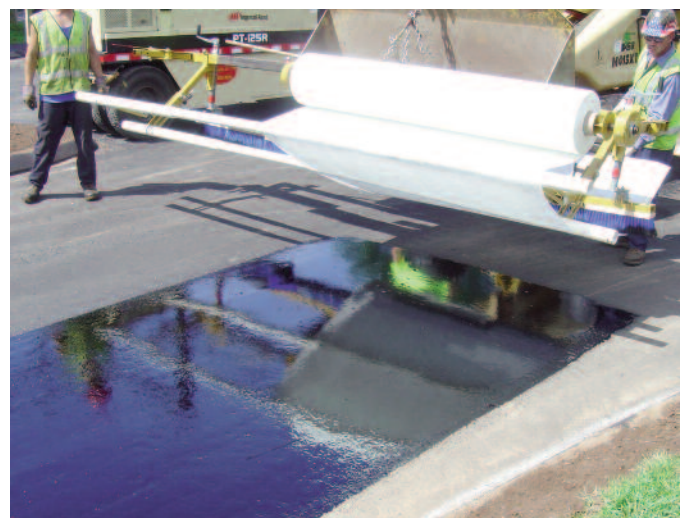
Figure 3: PG 64-22 asphalt tack applied and TruPave® installed.
