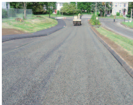
Figure 6: Stone rolled in-place to embed into TruPave.
