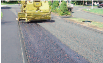
Figure 8: 2nd application of stone applied at 22 lb/sy.
