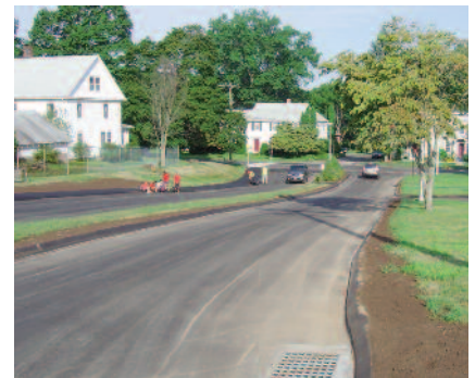
Figure 2: Reconditioned roadway surface.
