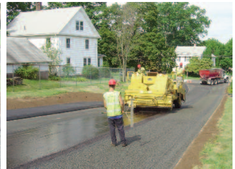
Figure 5: Emulsion applied over TruPave®-1st layering of stone applied.
