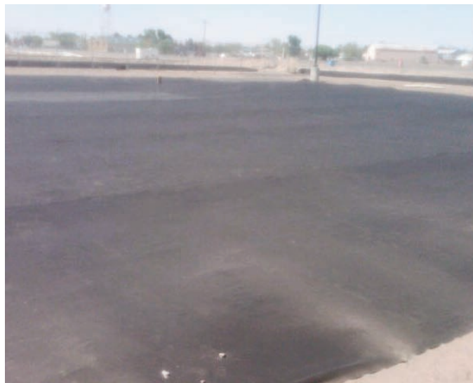
Installation of Mirafi® 160N in the landscape areas.
