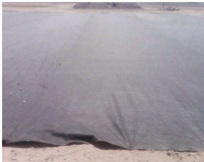
Installation of Mirafi® 160N in the landscape areas.
