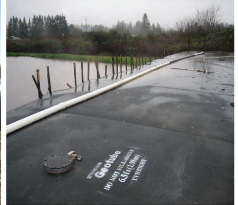
Figure 3. Filled Geotube® unit next to clean lagoon.
