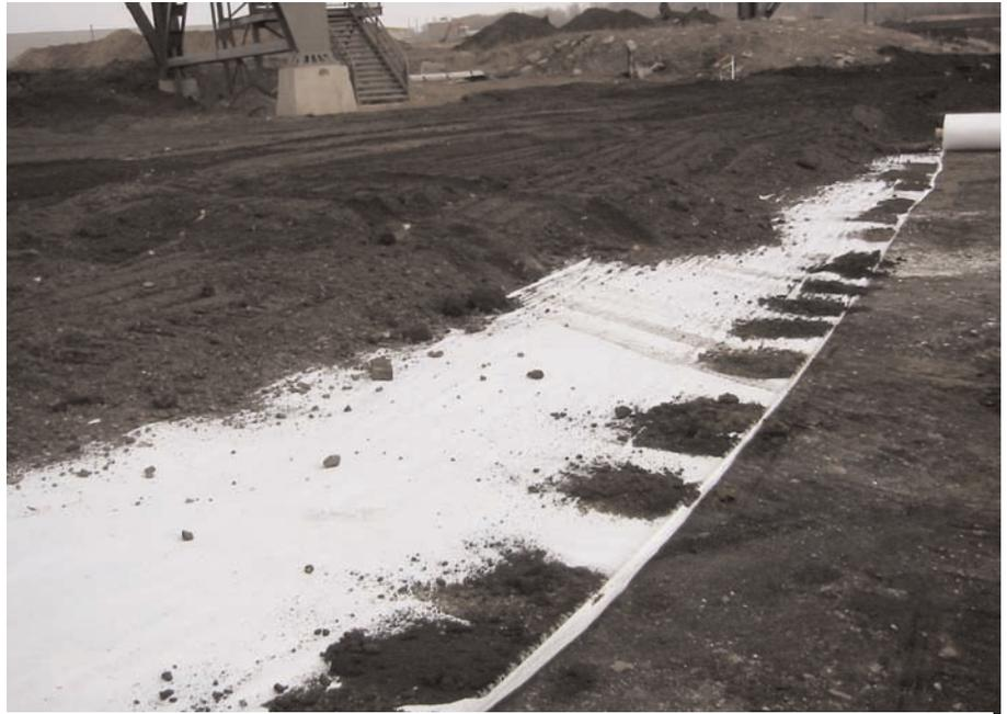
One foot of silty material was placed on top of the geotextile and compacted to 95%.
