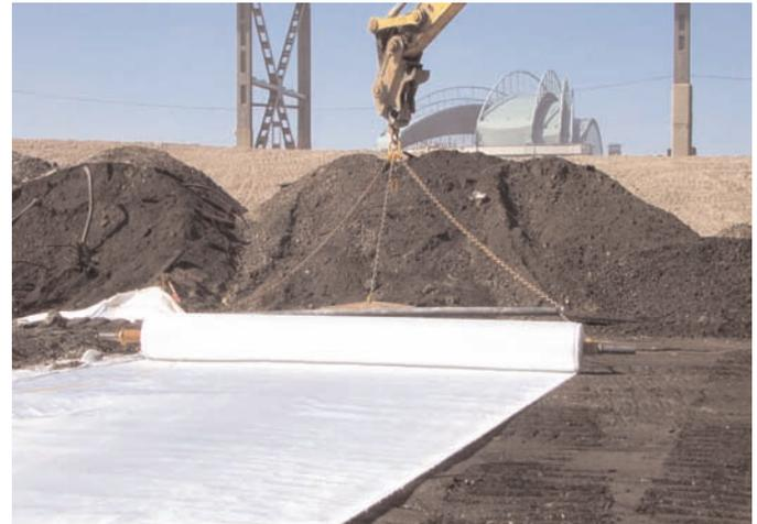
Large master rolls of Mirafi® HS800 were laid out in one continuous panel.
