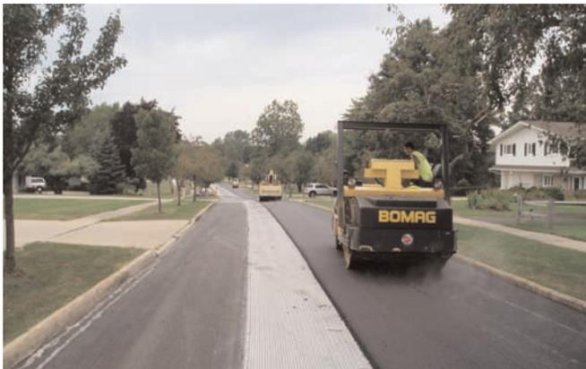
Compaction of polymer modified asphalt.
