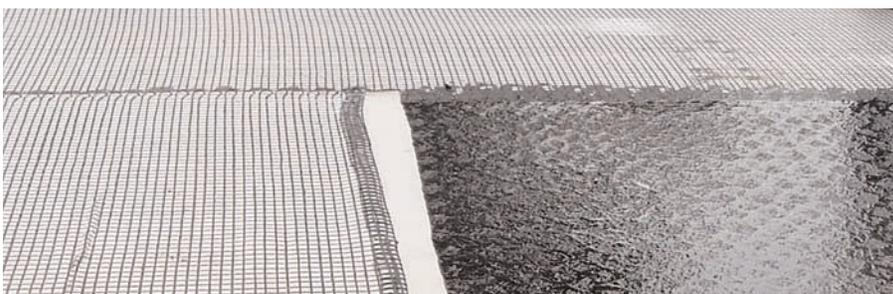
A tack coat of .23 gal/sy was used to form a moisture barrier.
