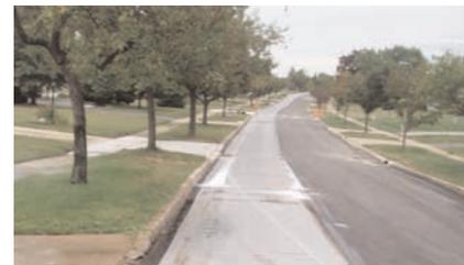
1in leveling course, Mirafi® FGC100 paving grid, 1.5in of compacted hot mix.
