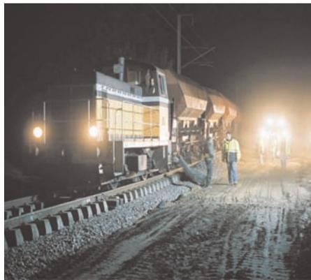
Installation of the GeoDetect® and ballast layers.
