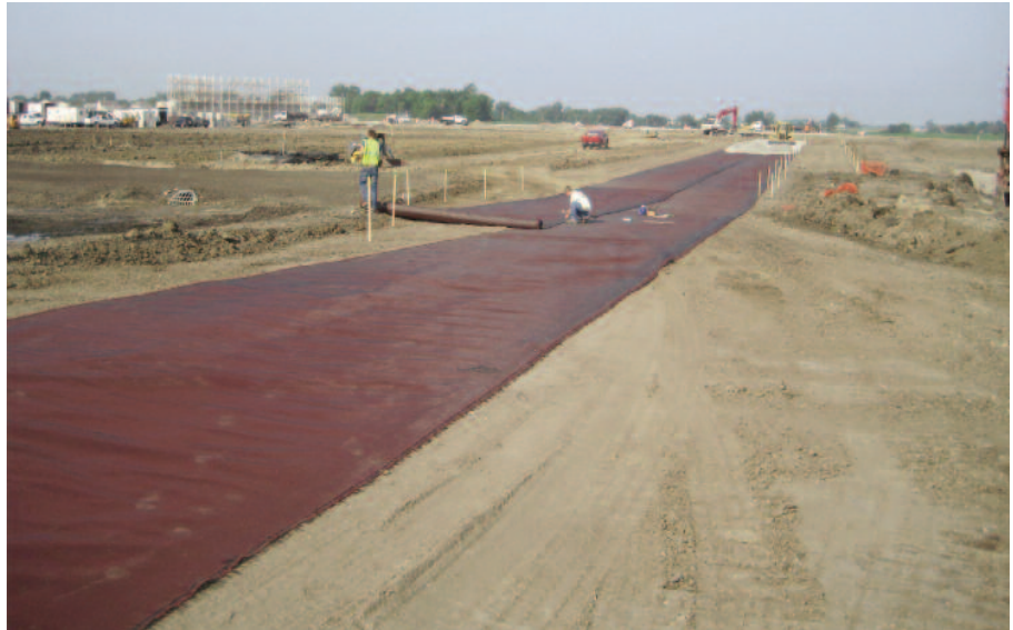
Mirafi® RS580i being installed over weak subgrade.
