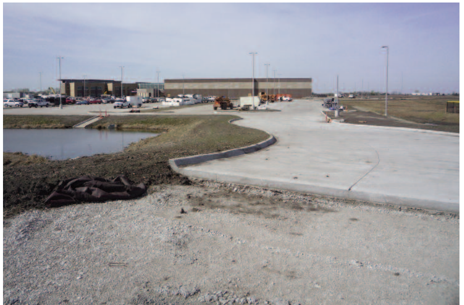
Concrete pavement installed over Mirafi® RS580i geosynthetic reinforced aggregate.
