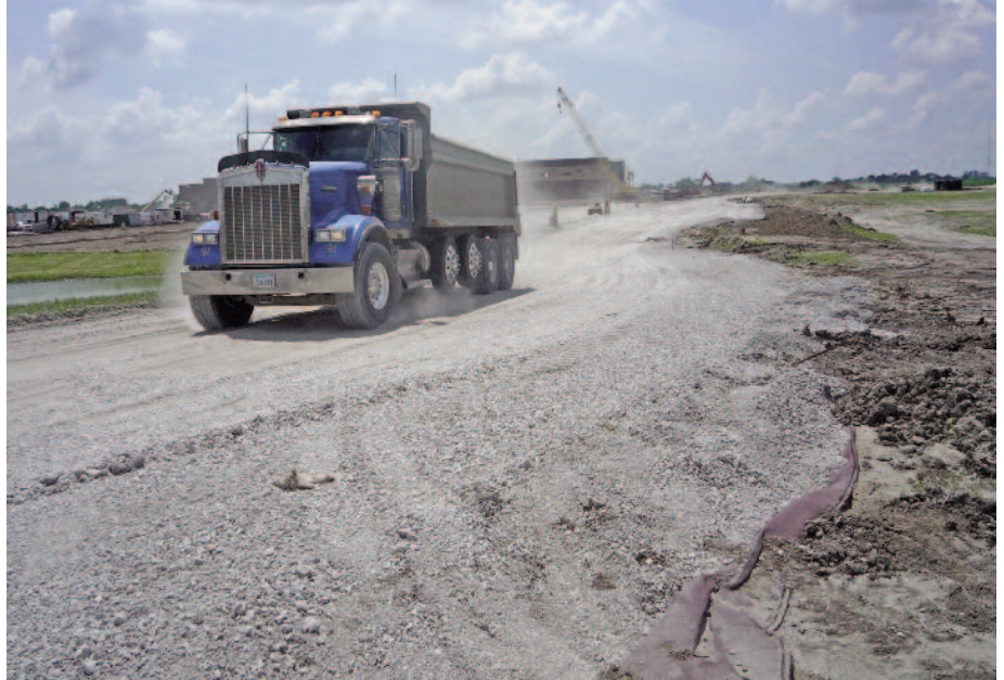
Access road supporting truck traffic.
