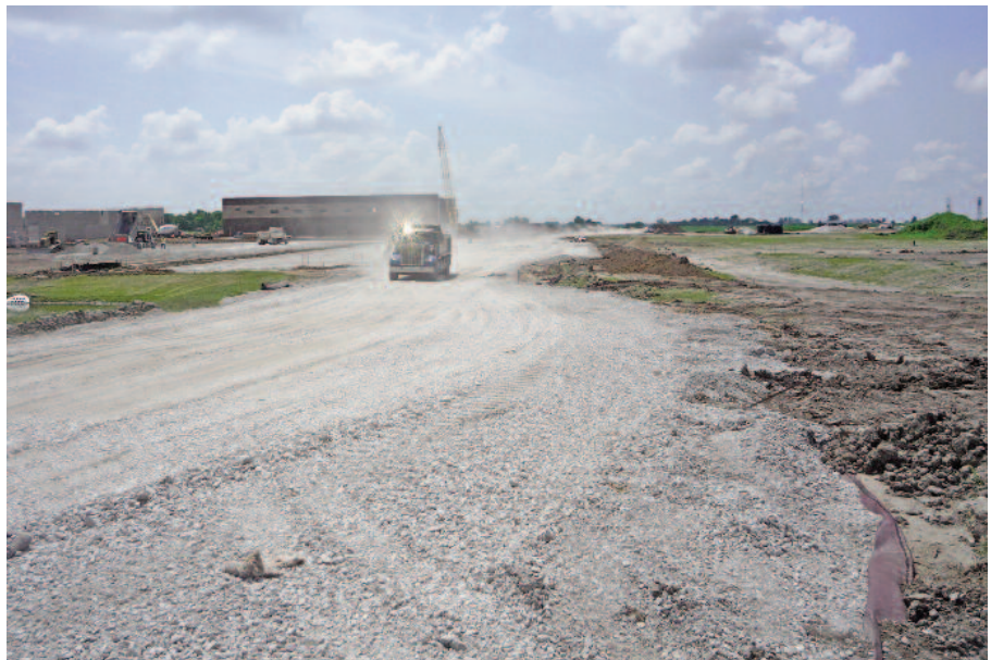
Installation complete with 6" aggregate.
