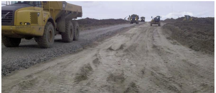
Haul road constructed with Mirafi® HP570 as designed.
