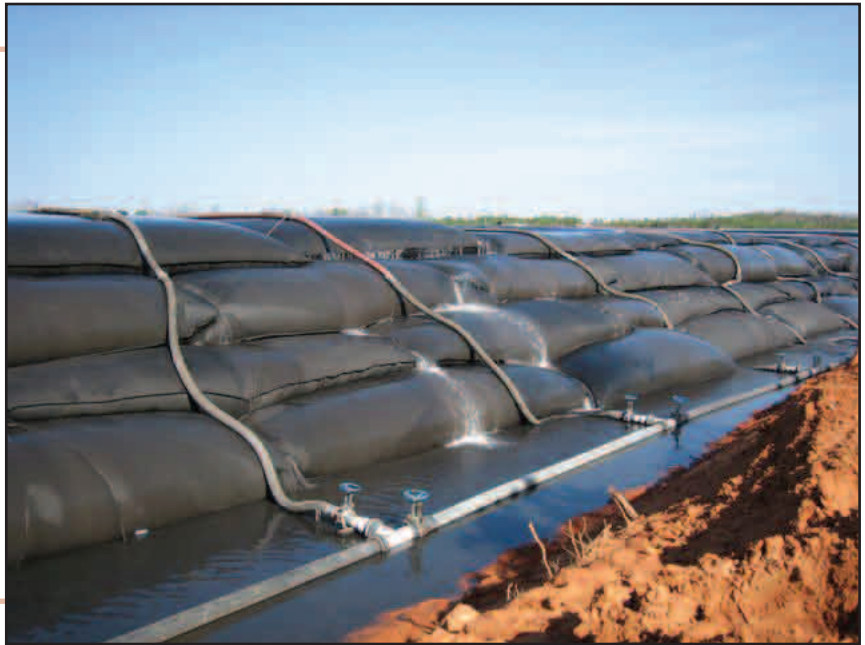
Geotube® Containment and Dewatering technology was used to dispose of slurry waste from North River Mine.
