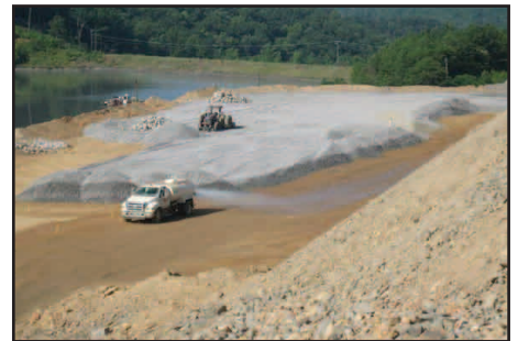
The site was prepared for the Geotube® containers.
