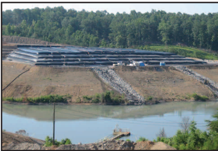
One 4-layer stack of Geotube® containers was buried before another four layers were placed and filled on top.
