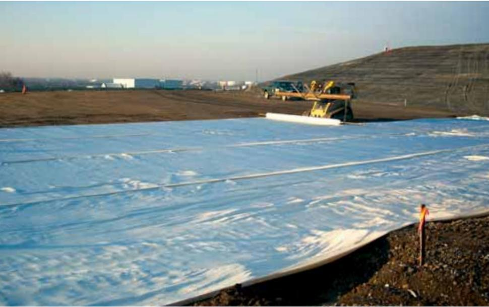
Installation of the first layer of high-strength geotextile.
