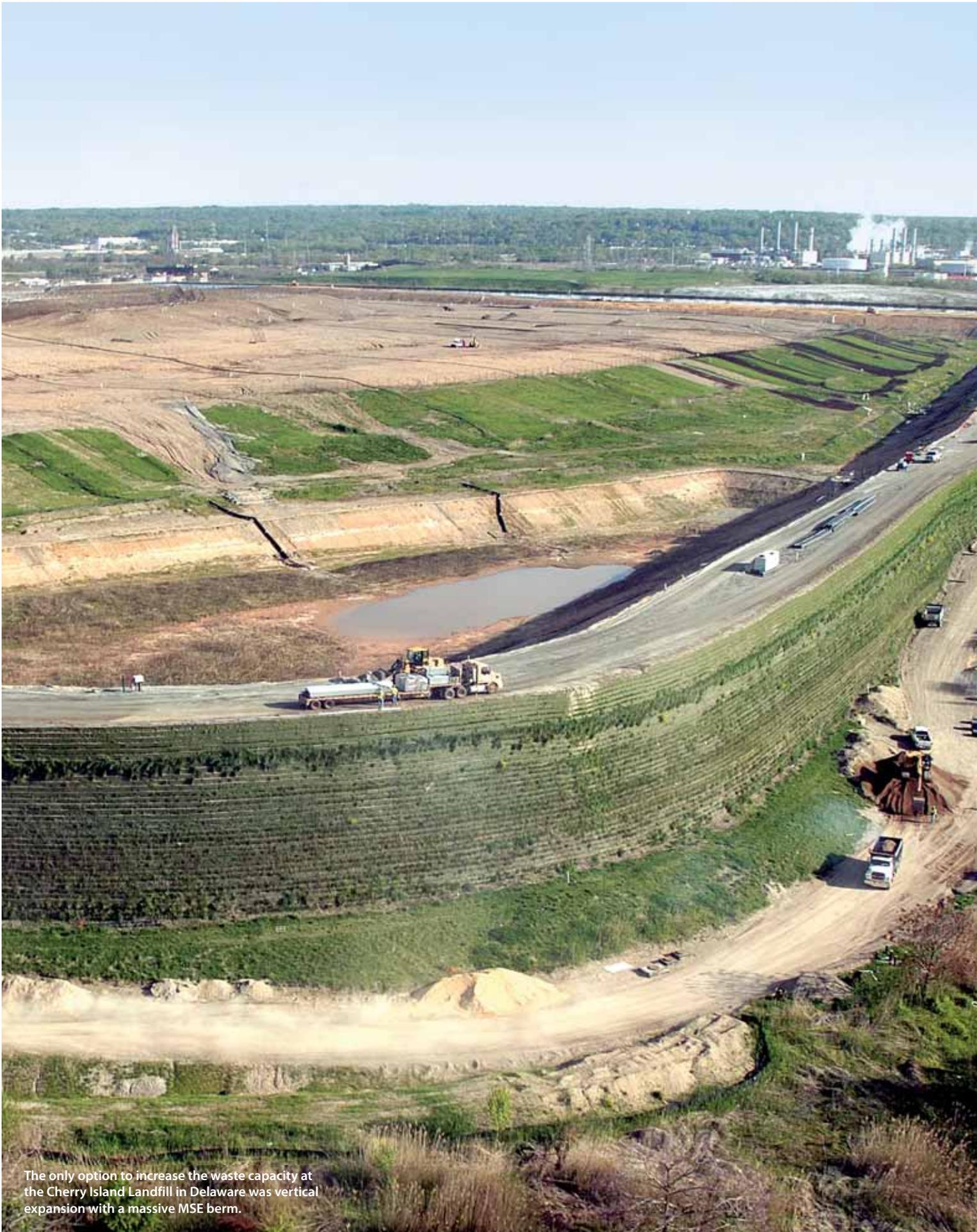
The only option to increase the waste capacity at the Cherry Island Landfill in Delaware was vertical expansion with a massive MSE berm.
