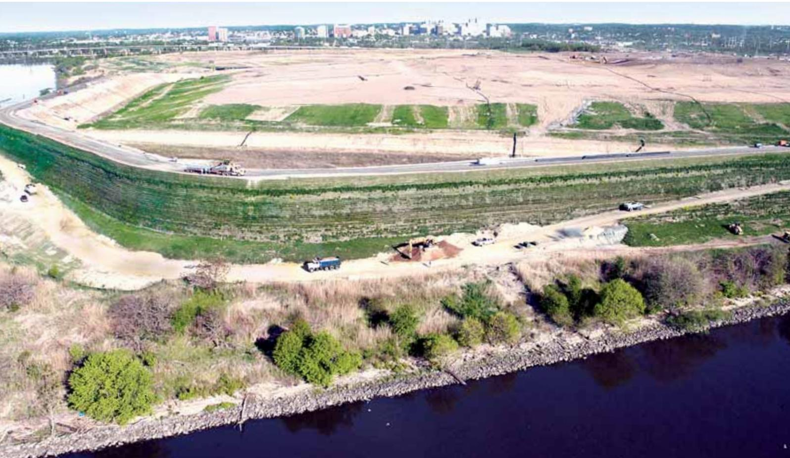
An MSE berm almost two miles in length was the critical component of this vertical expansion project. Located at the confluence of two rivers, the Cherry Island Landfill also presented challenging subsurface conditions.
