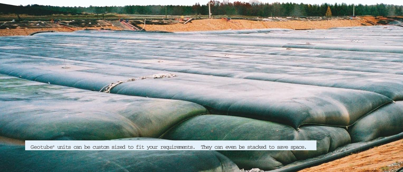
Geotube® units can be custom sized to fit your requirements. They can even be stacked to save space.
