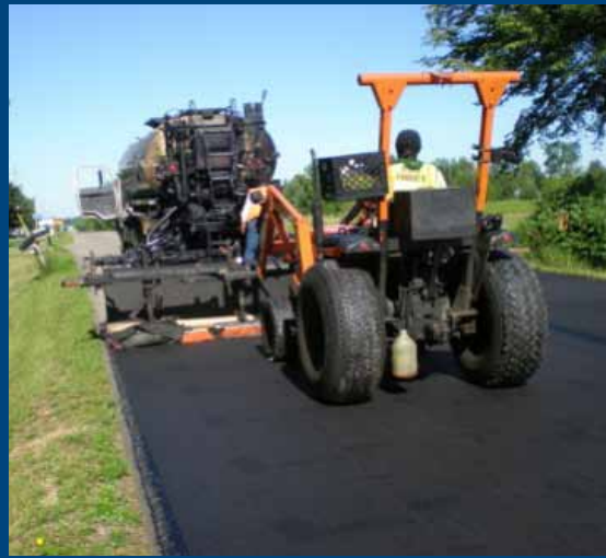
INSTALL FABRIC OVER LIQUID ASPHALT
