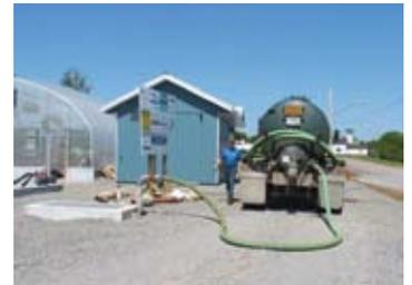
The Eganville wastewater facility features two outdoor dewatering cells and a cold-weather greenhouse enclosure for year-round use of Geotube dewatering technology. This accommodates winter emergency pumpouts.
