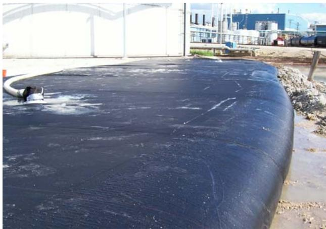
A 60' x 100' Geotube® was installed @ Site A to contain and dewater approximately 300,000 gallons of lagoon residuals.
