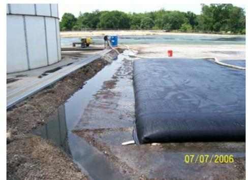
The 60' x 100' Geotube® containers @ Site B are pumped periodically to a height of 7' to dewater and consolidate 0.6 MG of lagoon solids. Clean filtrate water from the Geotube® container is collected from the lay-down area and returned to the headworks of the facility.
