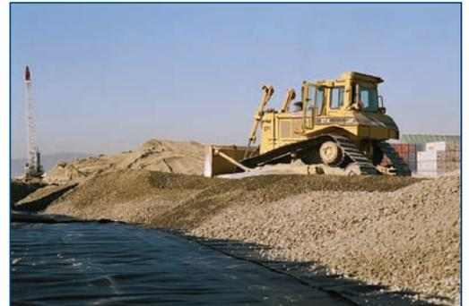
Mirafi® HP570 provides subgrade stabilization and base reinforcement.
