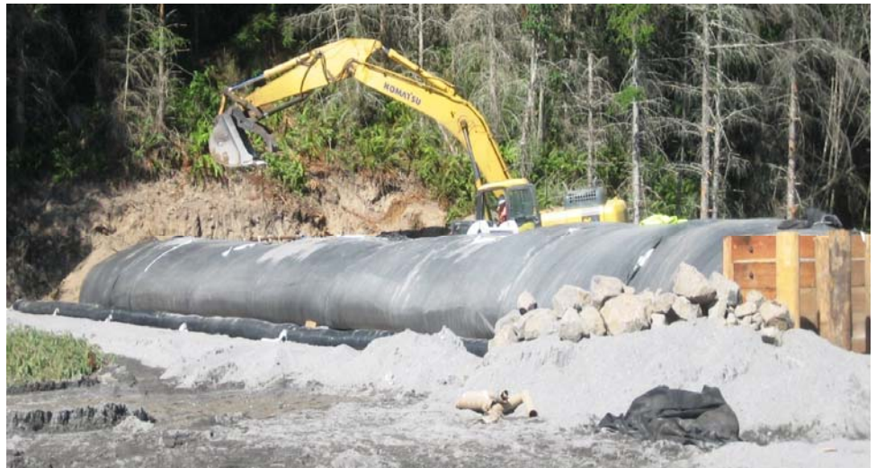
Geotube® Debris Shield encapsulating and protecting a Geotube® container from water-carried debris
