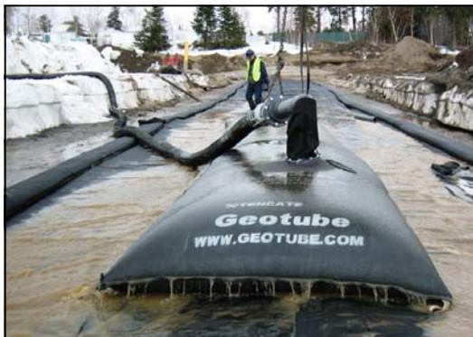
A Geotube® unit being filled with sand slurry mix as the jetty takes shape. Anchor tubes are visible on both sides of unit.
