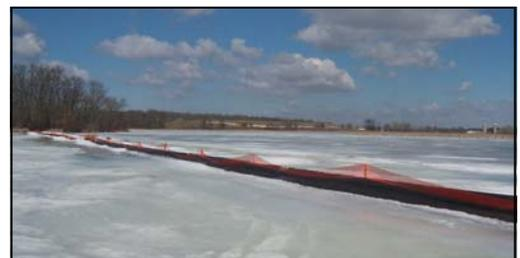
*Geotube® units remained in place despite the harsh Wisconsin winters and heaves of ice sheets.*
