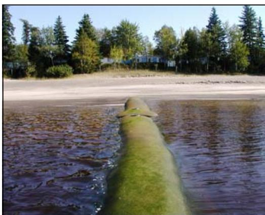
A view of the lake shoreline from a completed jetty. Marine growth can be seen on the Geotube® unit.
