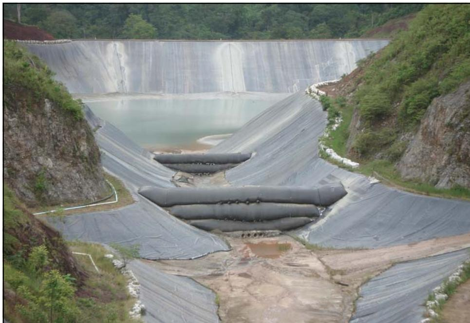
*El Mochito Mine, Honduras: Two Geotube® debris dams provide protection from potential landslides in the area of the tailings lagoon (top of the photo.) Geotube® technology offered many benefits: shorter installation time, lower installation costs due to using local fill materials, and the environmental liner remained in place.*
