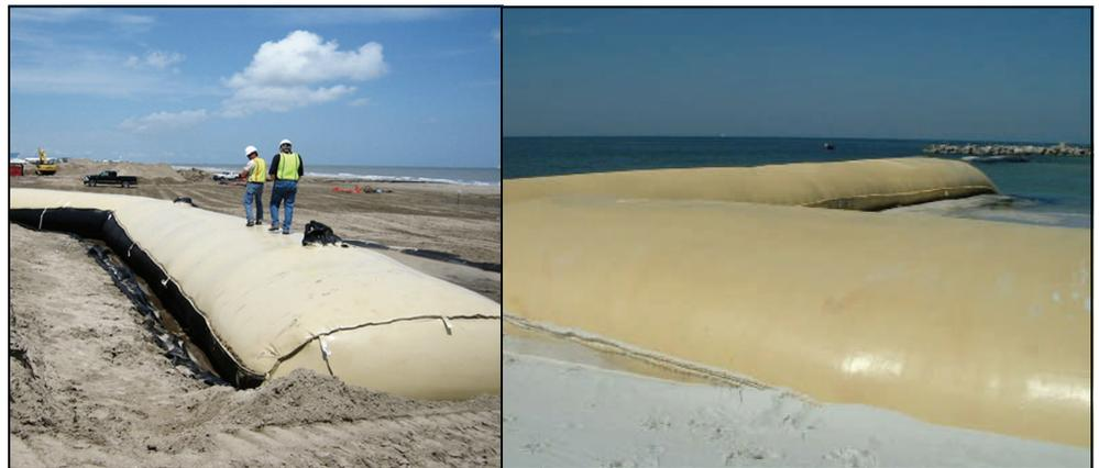
Multiple Geotube® installation sites have utilized the sand-colored polyurea coating. The advanced coating offers strength, longevity, and durability — as well as an aesthetically pleasing appearance on the beach.
