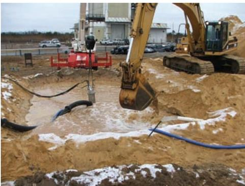
*Imported sand and water from the ocean and river estuary were mixed together in two slurry pits and pumped into the Geotube® units.*
