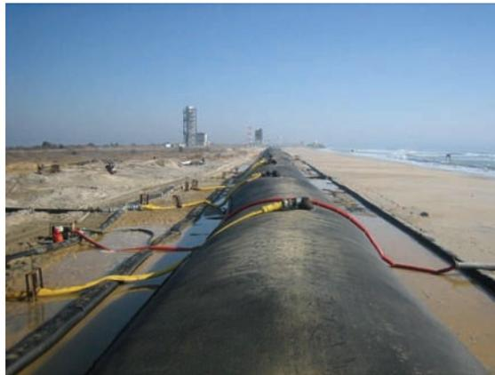
*A header system with multiple flexible lines fed the sand slurry into the Geoport™ filling ports.*
