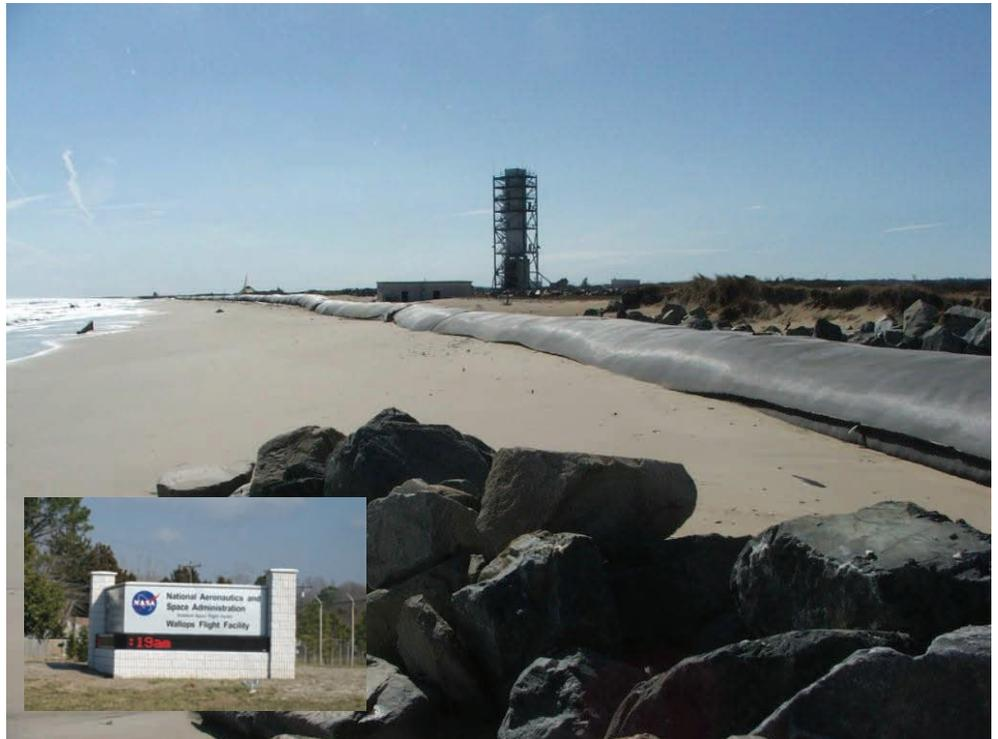
*A wall of Geotube® containers, 4,600 linear feet long and 6-feet high, was installed to protect NASA's Wallops Flight Center on Wallops Island, Virginia.*
