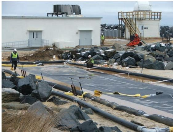
*Scour aprons were placed under each Geotube® container and secured with sand-filled anchor tubes.*
