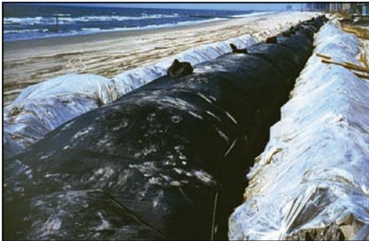
The Geotube® container will serve as the core of a sand dune when covered with sand and vegetated thus serving as a protection against storm surges.
