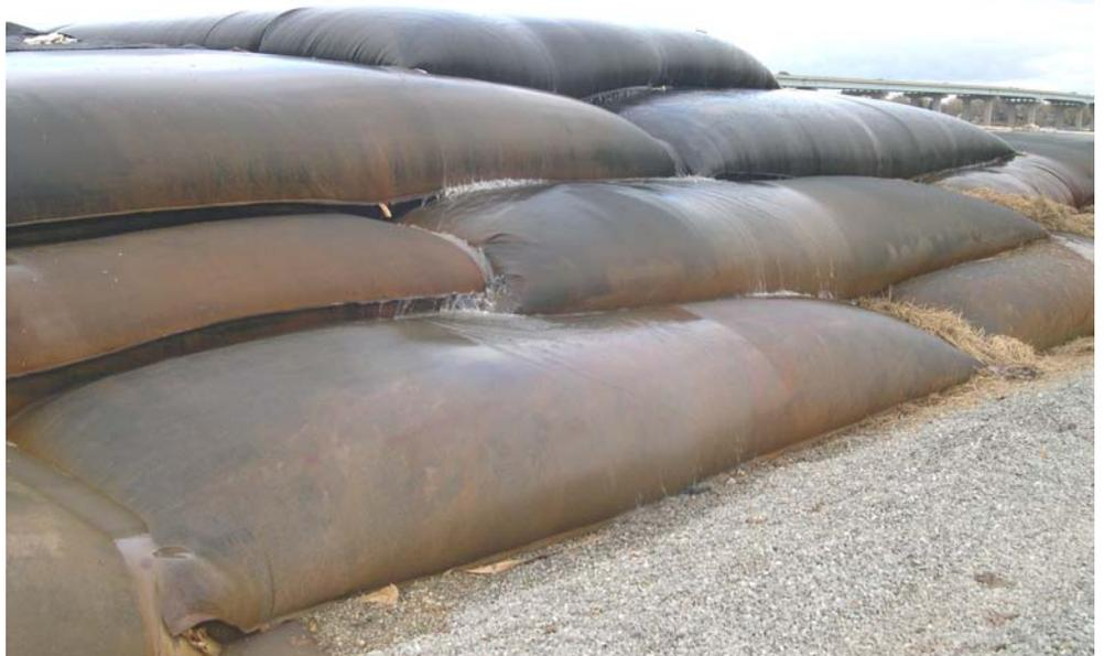
*Geotube® containers stacked in a dredging operation at Fox River. Geotube® dewatering containers can be layered like this to increase dewatering volume for the space allotted. For a large project, this can be critical.*
