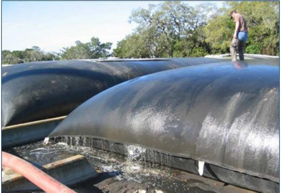
*In Jekyll Island, GA, Geotube® dewatering containers were used to provide a fast way to remove more than 400,000 gallons of sludge from digesters. The Geotube® containers fit into the facility's existing drying beds and made the process simple.*
