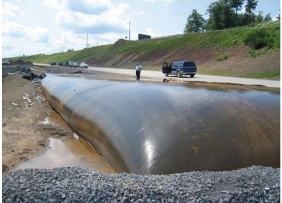
*Geotube® units being used at the I-99 site near Skytop Mountain, PA. Geotube® dewatering technology was used to contain heavy metals and other contaminants from pyretic rock unearthed during road construction. This prevented acid runoff problems.*
