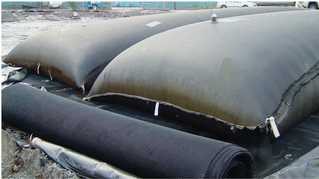
*Readily-available Geotube® MT units were used for the pilot project to gauge dewatering effectiveness.*
