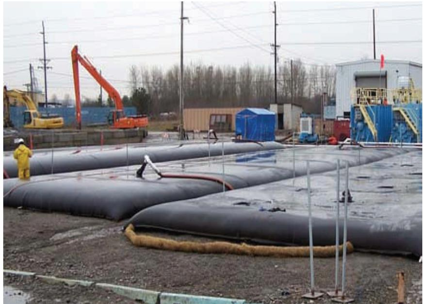
*Geotube® containers deployed at the Hylebos Waterway cleanup site. Three units were manifolded together. As one reached its designated fill height, the next unit would come online to provide uninterrupted dewatering.*
