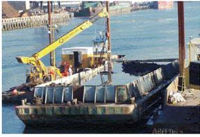
*Dredging was done using an articulated fixed arm dredge with a 3.0 cy (2.3 cm) closed hydraulic clamshell bucket.*
