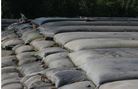
*Geotube® containers can be stacked several units high to increase dewatering capacity in a confined space.*
