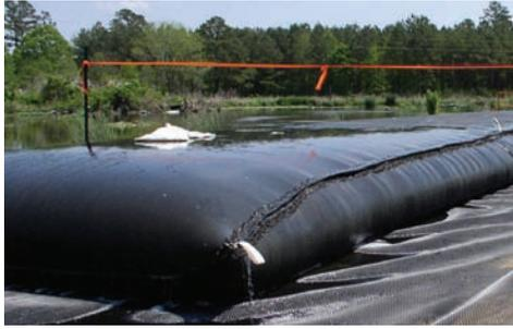
*A simple colored ribbon stretched over the top of a Geotube® unit can signal the operator when the unit reaches maximum pumping height.*
