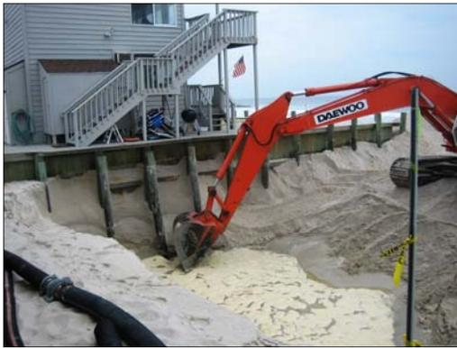
A 12' deep excavation was required to achieve the designed final dune elevation.
