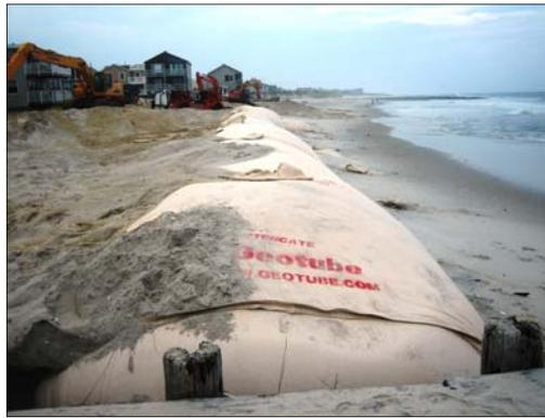
Geotube® unit unique flat ends abutted the piers on either end of the installation making a tight fit. Tri-State Dredging placed and filled the seaward tube, then the dune-side tube. Upon completion of the first layer, the final 200' long Geotube® container was stacked on top and filled to six feet.
