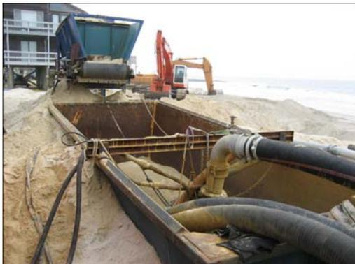
Sand to fill the tubes was imported, then scurried with sea water in a 30 cy roll-off box to be pumped to the tubes. Tri-State Dredging used a 6" submersible hydraulic pump to fill the Geotube® containers..
