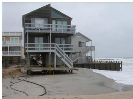
Before Geotube® container protection, this house was being undermined. The beach was gone.
