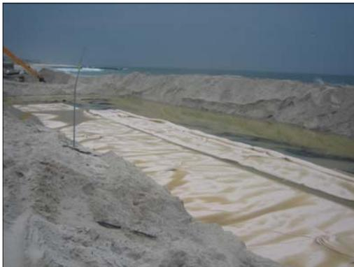
Scout aprons were deployed and anchor tubes filled before placing the 34' circumference x 145' long seaward tube. The challenge for the contractor, Tri-State Dredging, was working around the tidal fluctuations.
