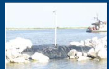
Installed plate for monitoring settlement
