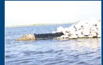
1x4 aggregate and 2,200 lb. rip rap with Mirafi® FW404 used as a separation geotextile
