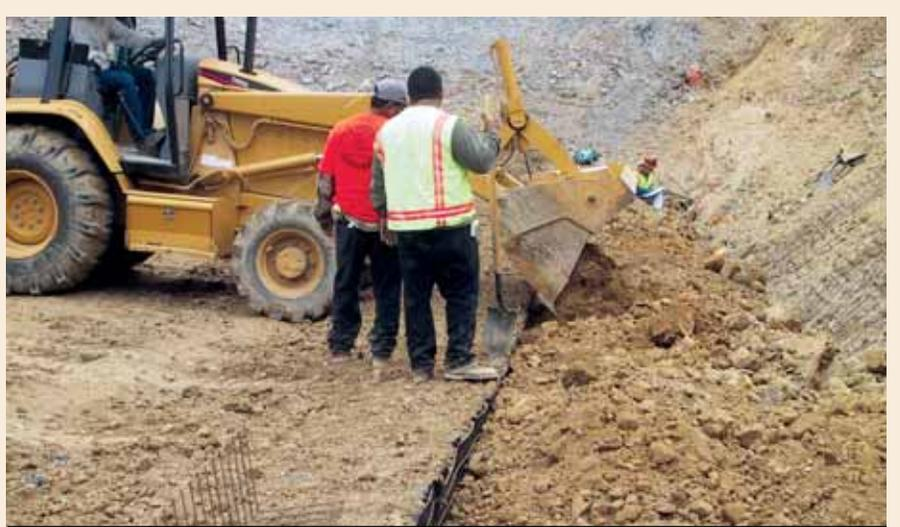
**Photo 4.** Constructing the geosynthetic-reinforced MSE wall buttress.
