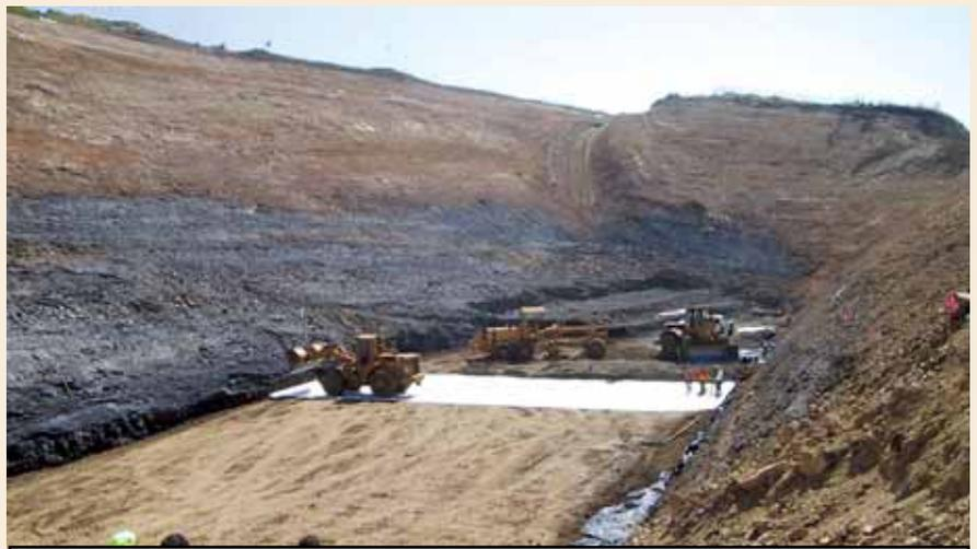
**Photo 3.** Numerous geotextiles and soil baskets provided vital internal support for the refilled hole.
