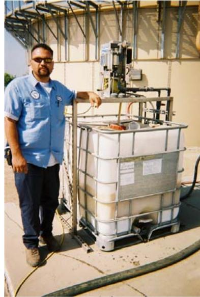
Raudel Juarez insures the polymer system is ready when sludge is transferred to the Geotube<sup>®</sup>
