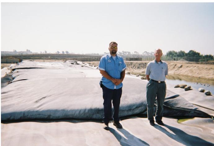
Raudel Juarez and Kelly Polk, district manager, stand in front of a Dewatered Geotube<sup>®</sup> that was eventually filled to a height of 5 feet. Solids inside the Geotube<sup>®</sup> feel like hard clay when walking on the dewatered Geotube<sup>®</sup>.
