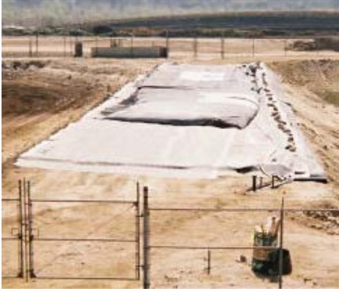
45 ft C x 43 ft L Geotube<sup>®</sup> is laying on a MCF-1210 ground cover which captures the clear filtrate to flow back to the headworks.
