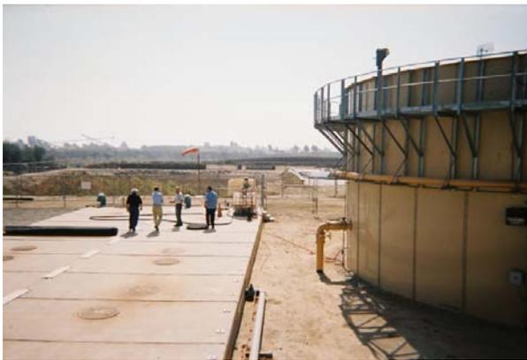
Saticoy Facility showing large septic tank now operating as aerobic digester prior to going to Geotubes<sup>®</sup> seen in background.
