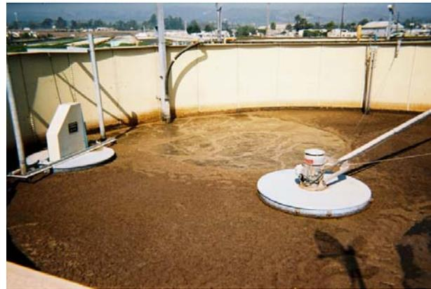
Two large circular tanks operated in batch mode provide alternating aerobic, anoxic, and clarification treatment of the wastewater.
