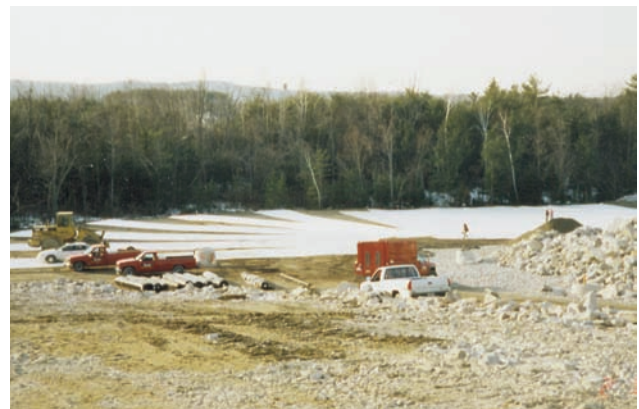
The first layer of HS2400.
