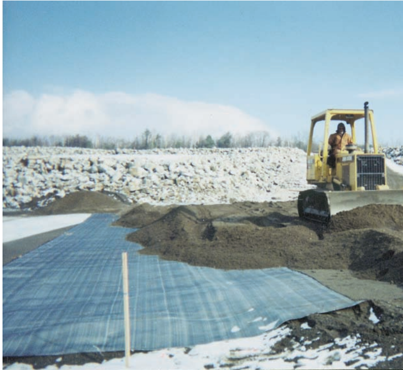
Backfill over the HS4200.
