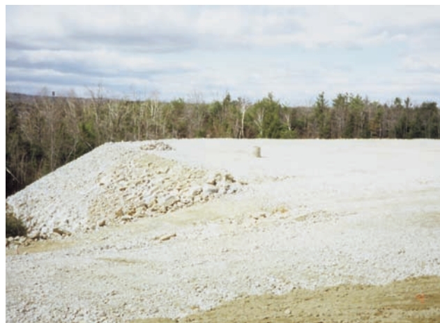
The completed 1:5:1 reinforced embankment.
