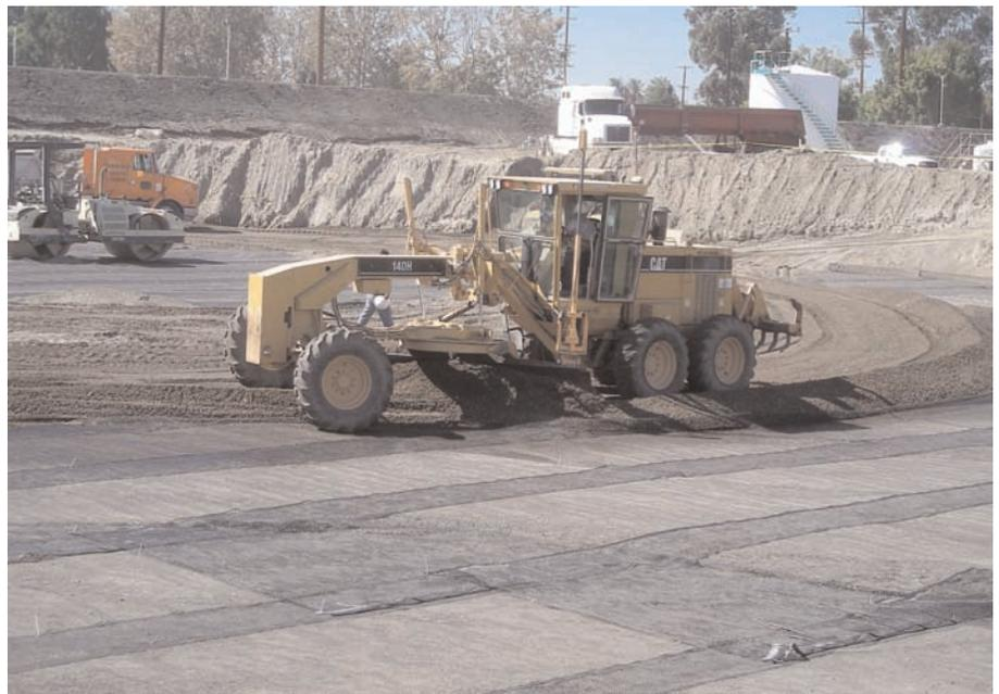
Rubber Tired Grader driving directly on the Mirafi® BXG12 geogrid.
