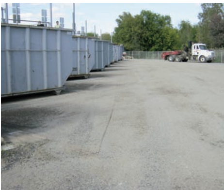
After completion of the work.
