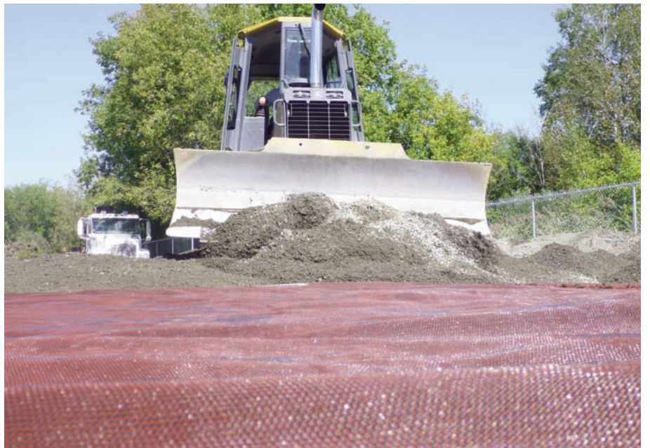
Placement of granular backfill on Mirafi® RS580i.
