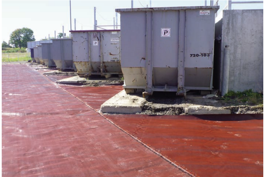
Installation of Mirafi® RS580i in front of the containers.
