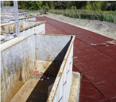
Installation of Mirafi® RS580i in front of the containers.
