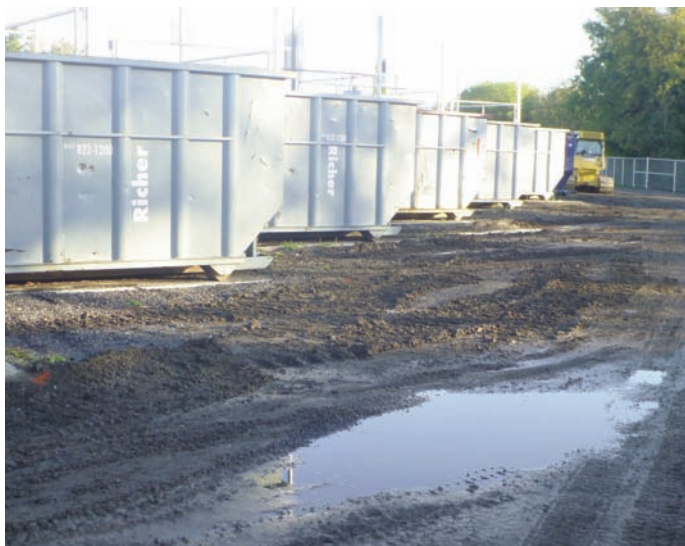
Site prior to excavation
