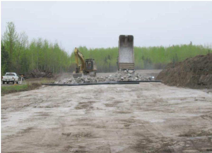
Proof rolled subgrade and rock placement.
