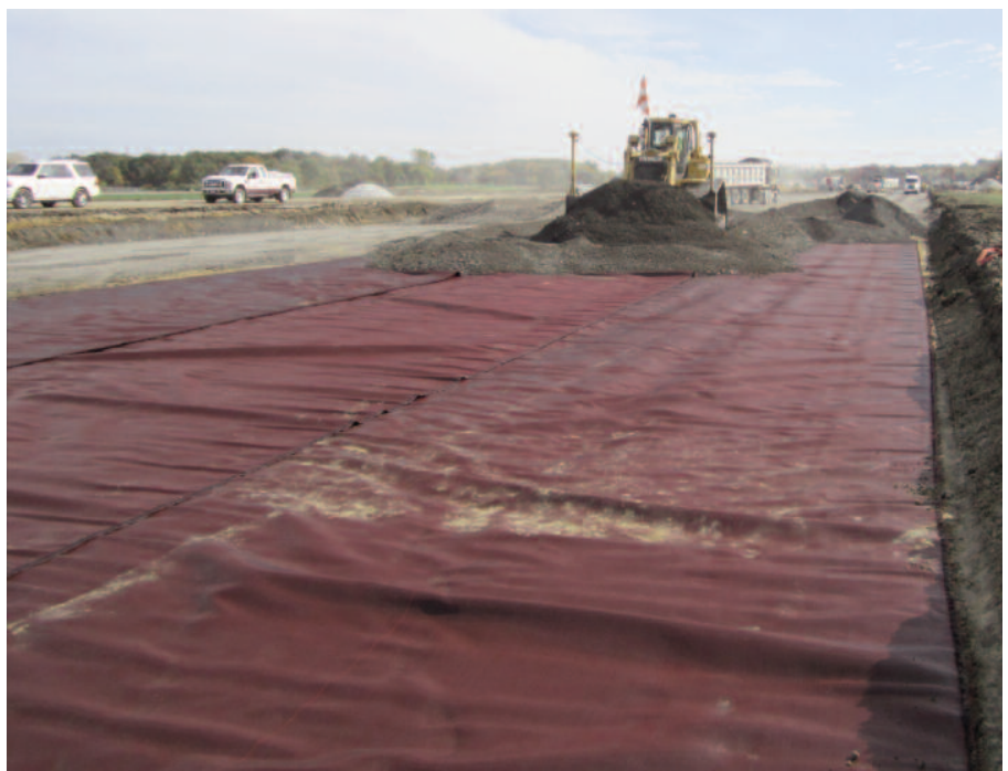
Bulldozer spreading the aggregate.
