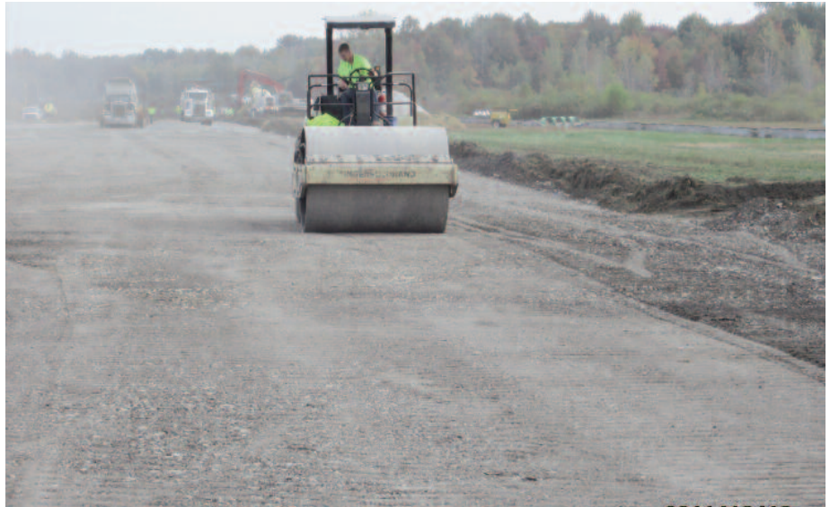
Section during compaction.
