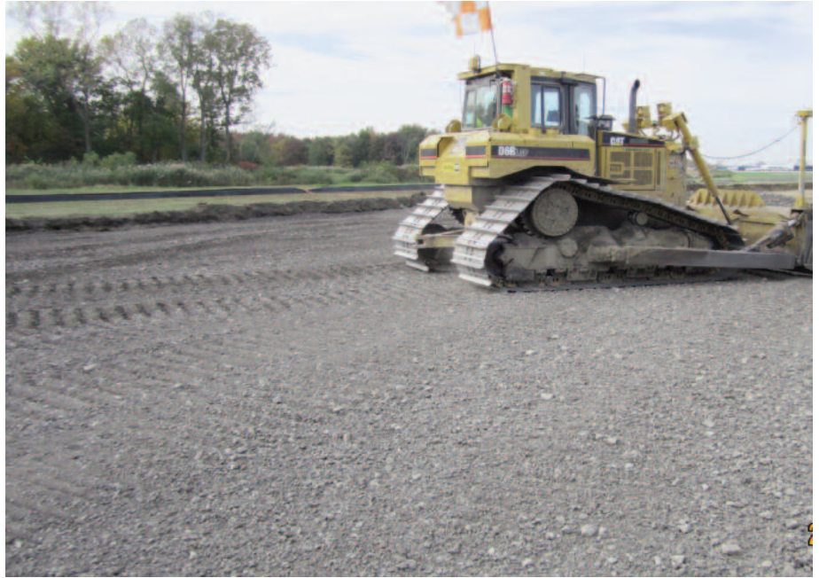
Section after placement of aggregate.
