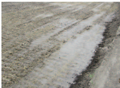
Taxiway area prior to subgrade treatment.
