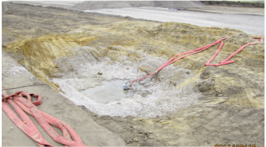
One of several dewatering sumps installed through out the site.
