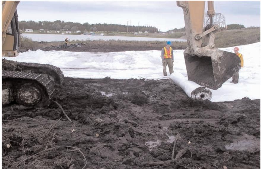
Using an excavator and a backhoe, the installer placed the panels directly onto the subgrade with a 1000mm (39 in) overlay at the joint between adjacent panels.
