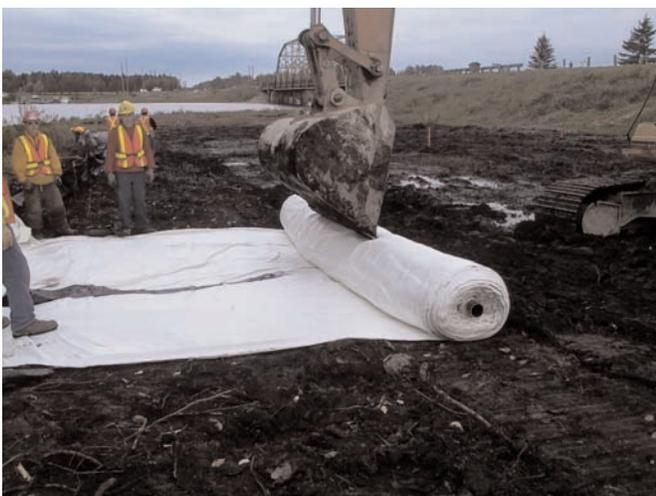
The design originally specified a geogrid with LTDS of 200N/m. Instead of multiple geogrid layers, one layer of Geolon® PET 600/100 was the ultimate solution.
