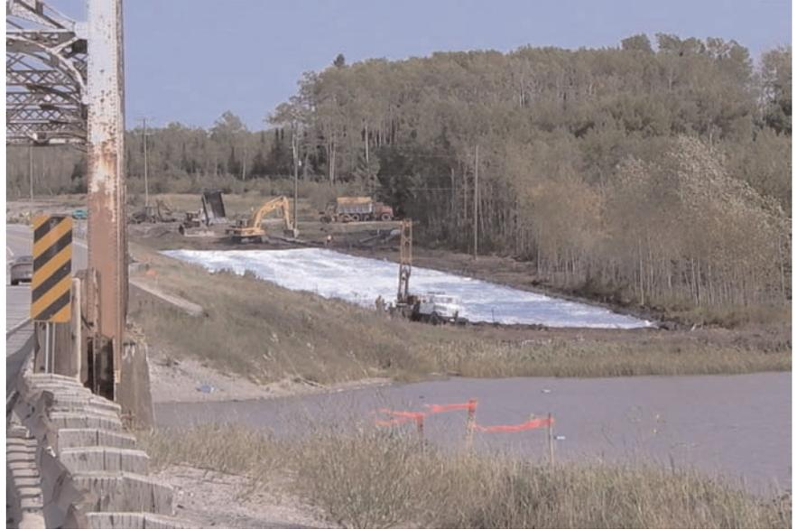
The largest area covered was 190m x 30m (623ft x 98ft) and was installed using nine sewn panels in less than a day.
