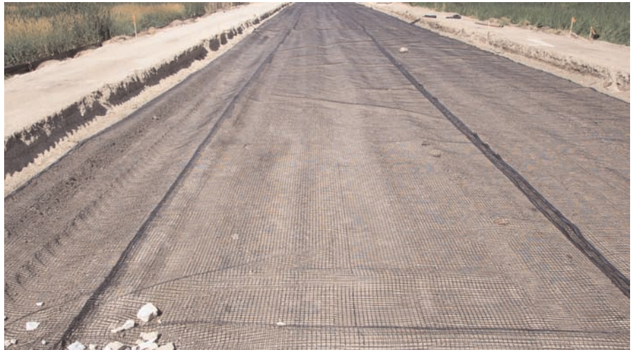
The Mirafi® BXG11 geogrid was rolled out in three sections.
