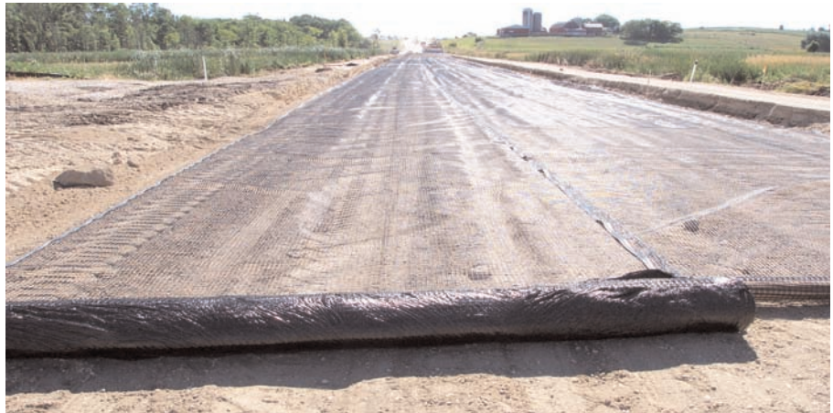
37,000 SY of Mirafi® BXG11 was required to reinforce the soft subgrade.
