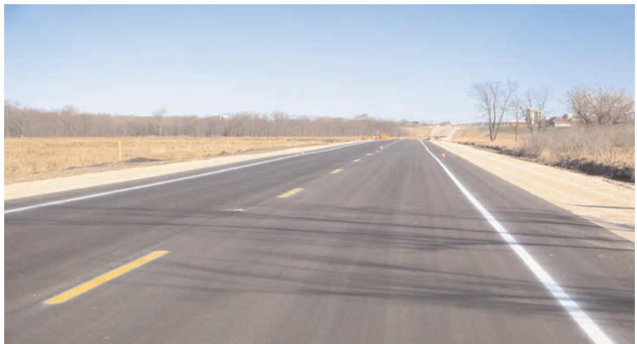
The completed highway. The project engineer saved $100,000 by using Mirafi® BXG11 on this roadway design.
