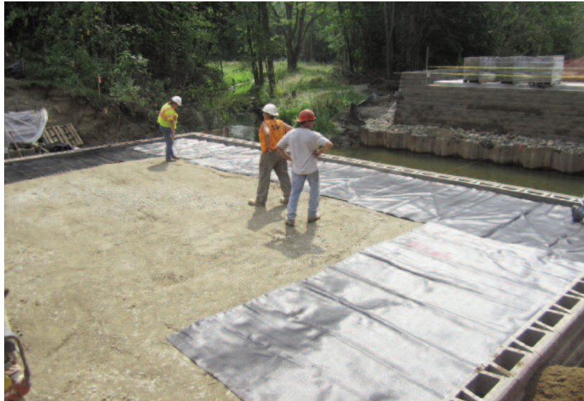
The cut Mirafi® HP570 placed behind the block.
