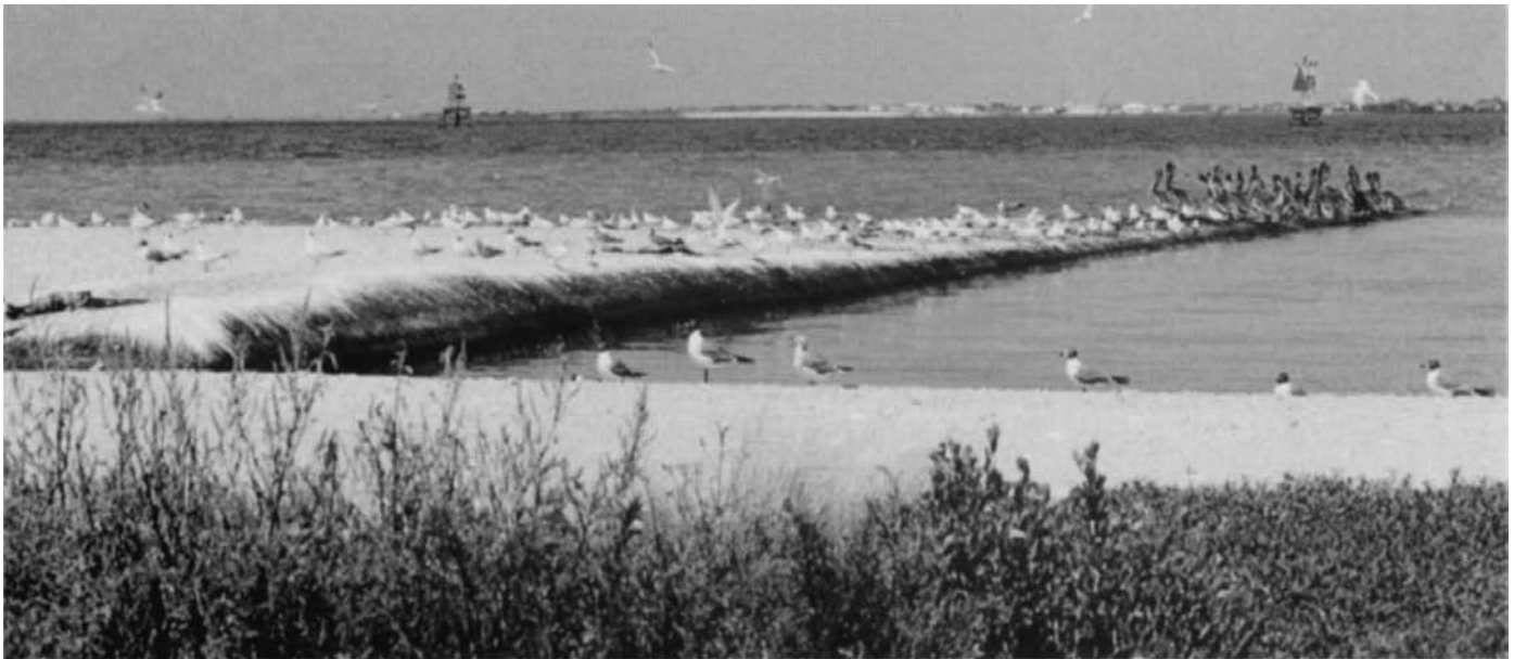
Geotube® six months after installation.
