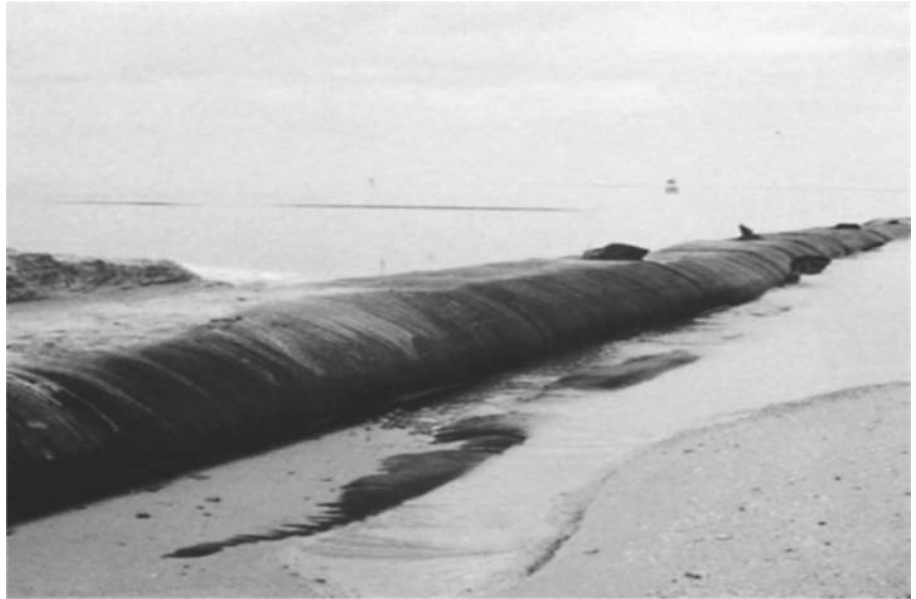
Installation of Geotube® containers and scour apron.
