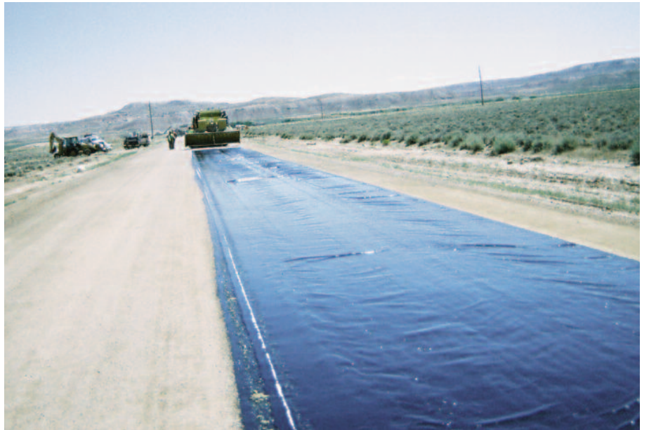
Figure 5: Emulsion applied over TruPave® & first layering of stone applied
