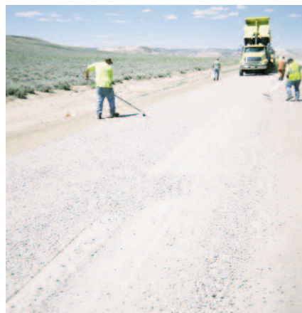
Figure 2: First layer of stone applied to TruPave® Mat.
