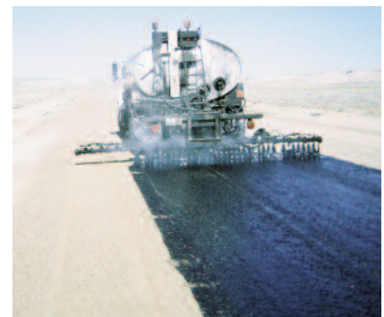
Figure 3: PG 64-22 Asphalt tack coat applied.
