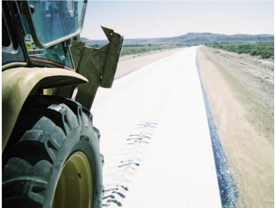
Figure 4: TruPave® installed over PG 64-22 tack application
