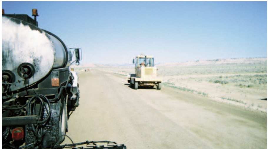
Figure 1: Road base preparation.
