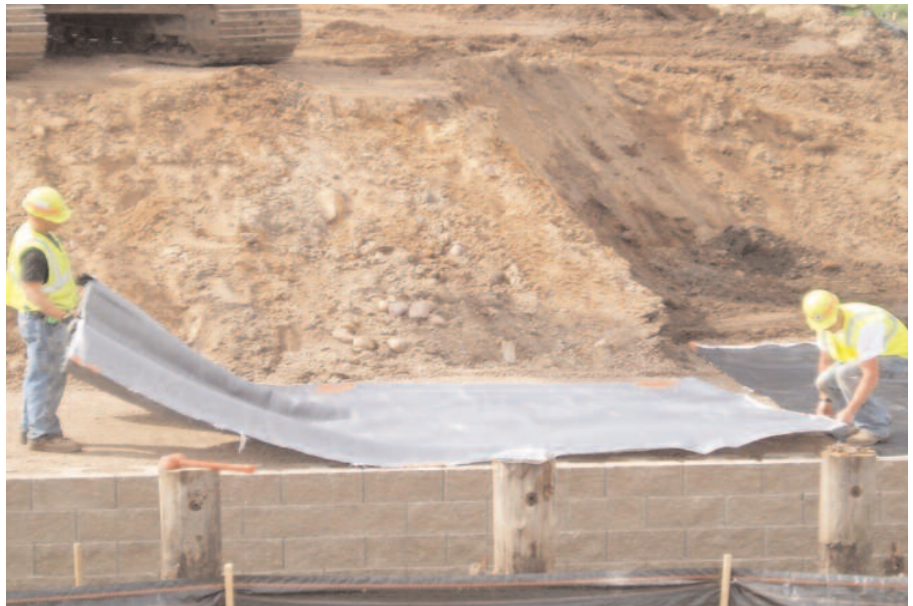
Placing the Mirafi® PET770 reinforcement layer.
