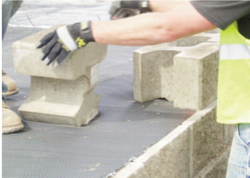
Hand placing the precast block.
