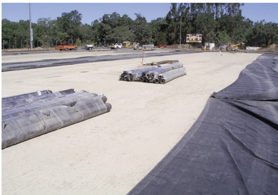
The convenient tri-pak packaging of Mirafi® HP270 made deployment at the jobsite quick and efficient.
