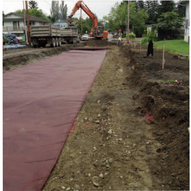
Above pictures: Mirafi® RS580i being installed over soft subgrade with the addition of crushed rock over the geosynthetic. This subgrade provided full width reinforcement across the roadway.
