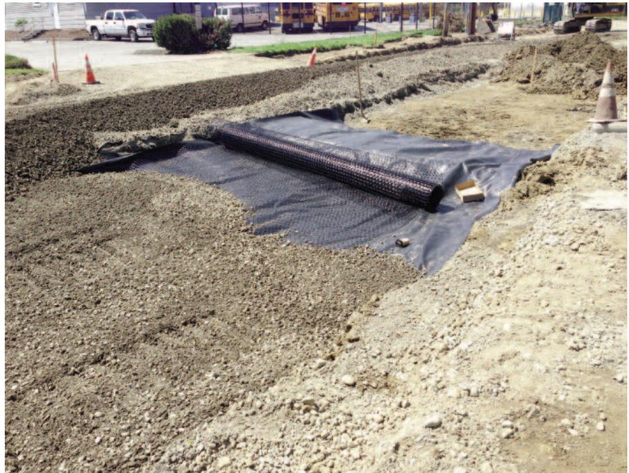
Installing crushed rock subgrade over mismatched sizes of fabric and geogrid.
