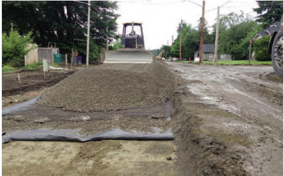
Installing crushed rock subgrade over mismatched sizes of fabric and geogrid.
