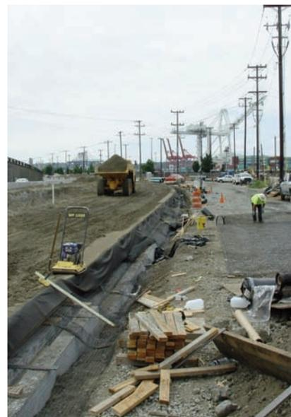
Beginning of wall construction using Miragrid® geogrid for reinforcement and face wrap.
