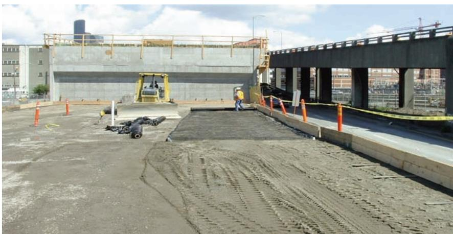
Wood forms are used to achieve compaction at the face of the wrapped face wall.
