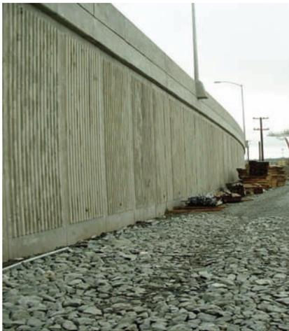
Finished wall with concrete panels attached to the fence.
