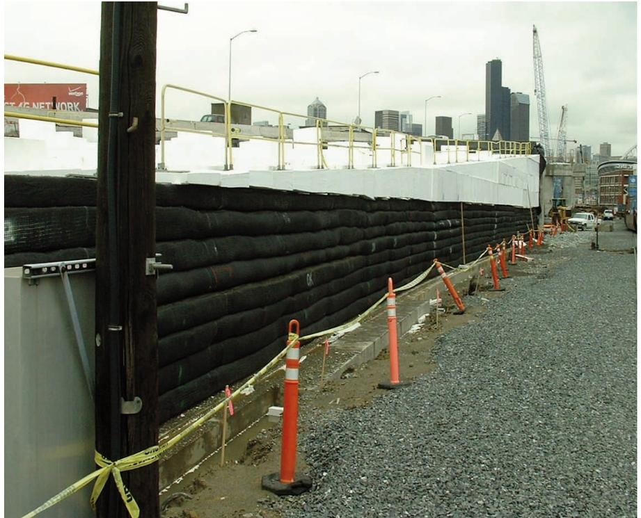
Completed seismic wall prior to placement of the concrete panels.
