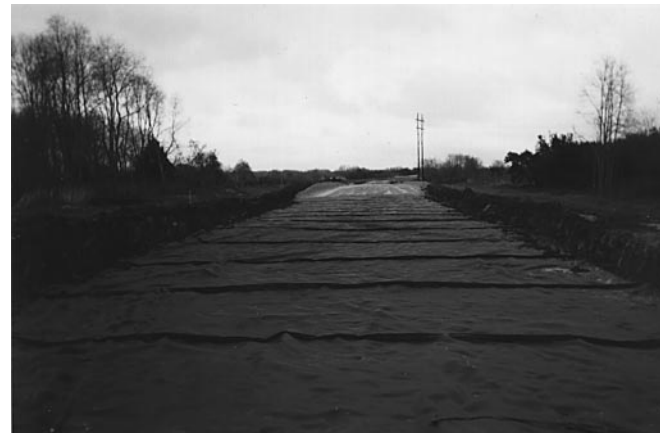
Deployment of geotextile allows construction
