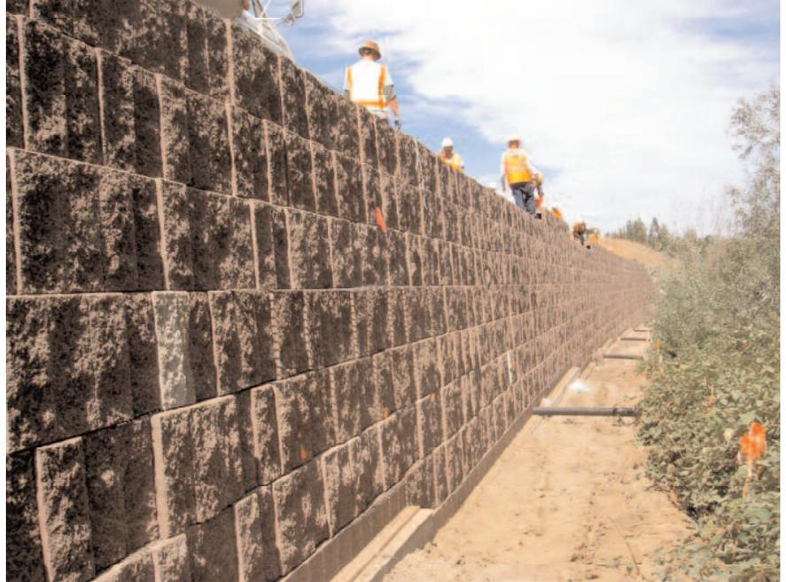
Partial completion of the Caltrans approved Anchor Landmark Wall with Miragrid® geogrid.
