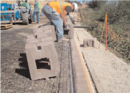
Setting the Anchor Landmark Wall Block unit and Miragrid® geogrid reinforcement.
