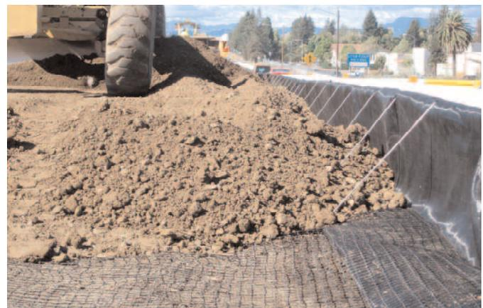
Native soil backfill is placed in temporary wirewall.
