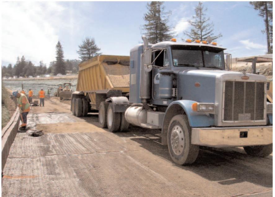
Installing MSE wall backfill over Miragrid® geogrid.
