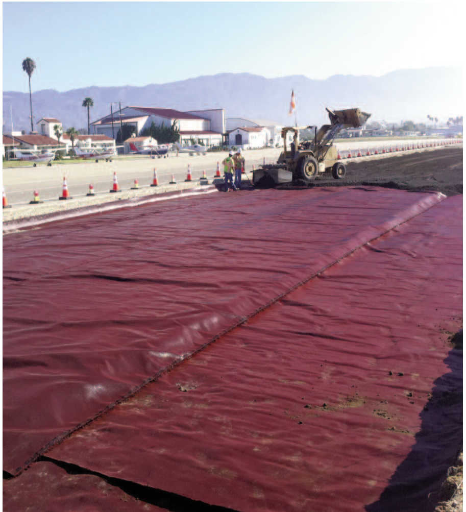
TenCate Mirafi® RS380i is laid out over the runway section at the Santa Barbara airport.
