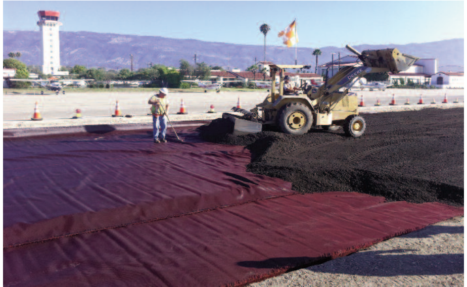
The bulldozer spreads out the asphalt grindings over Mirafi® RS380i.
